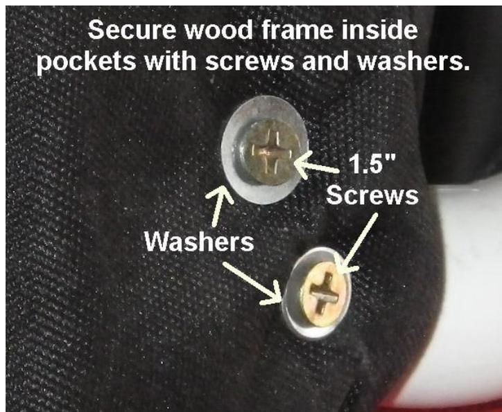
*The wood frames are screwed firmly to the pockets by running long drywall screws through the heavy pocket exteriors and into the 2x2 frame. Note the use of metal washers to avoid having the screw heads go through the pocket material.*
